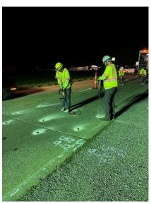
Linfield, Hunter & Junius, Inc. (LH&J) is providing resident inspection services for this project that consists of the replacement of existing concrete pavement roadway panels, milling and overlaying of asphalt shoulders, slab-jacking of existing concrete roadway panel and pavement striping along US 90/US 167 between the railroad crossing and E. Pinhook Road and along US 90 between LA 92 and LA 88. Duties include:
